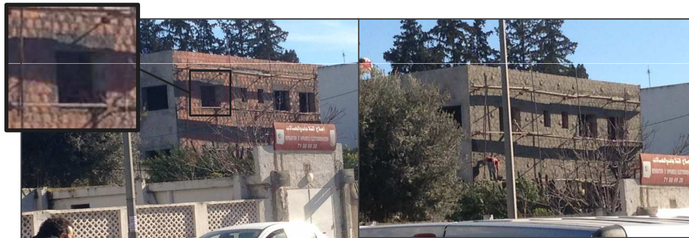
JUMELAGE Eco - Construction
