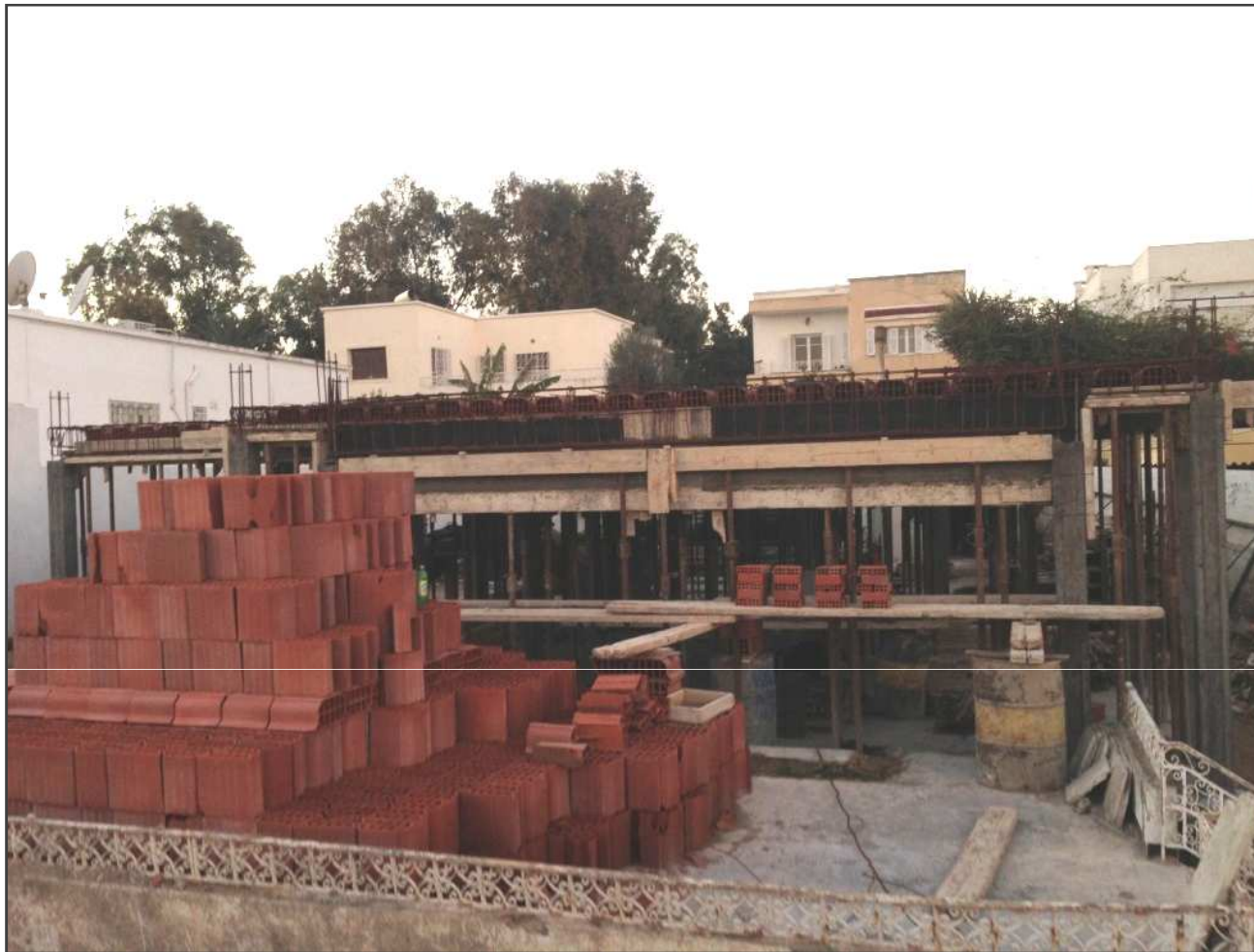
JUMELAGE Eco - Construction
