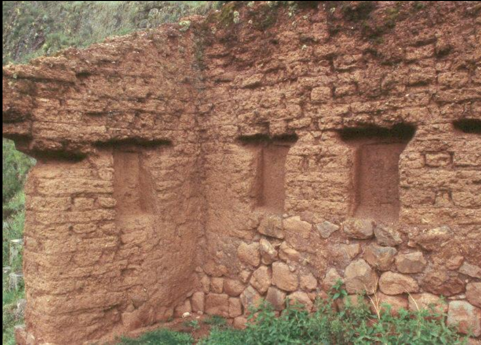
construction Inca, Pérou
