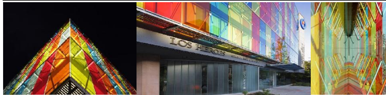
Los Heroes Building (source: popavenue.com)
